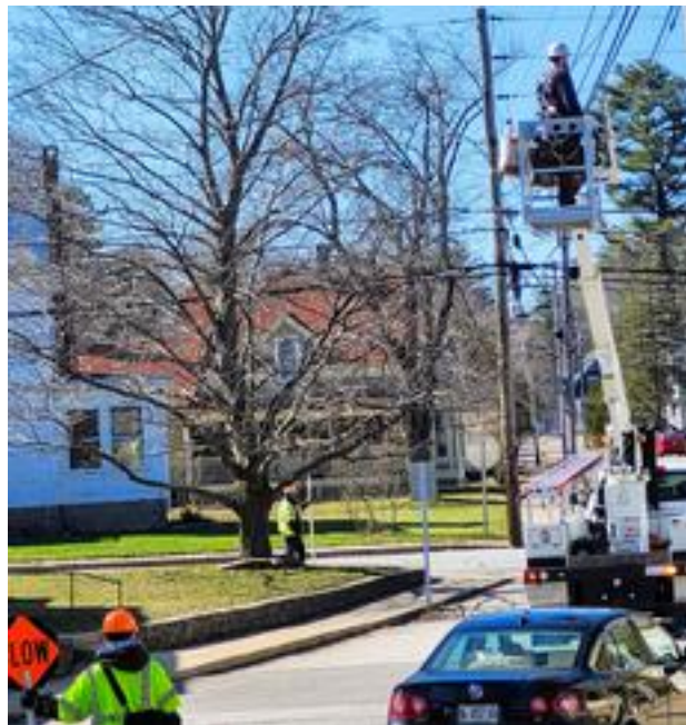
Crews for Breezeline string cable in Springvale. Photo: Lee Burnett
