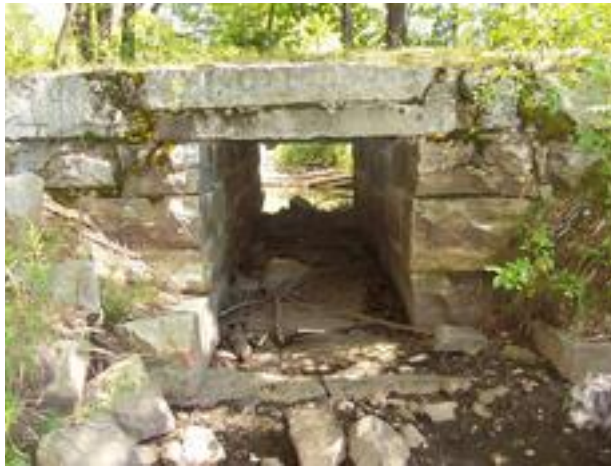
Cattle crossing along Sanford Rail Trail. Note the flat stones placed to aid cattle footing.
