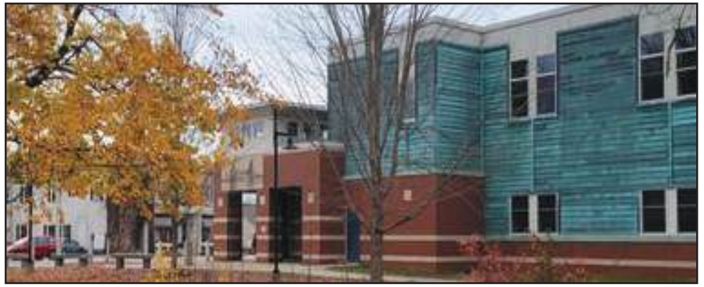
Springvale District Courthouse is on the way to being remodeled as apartments. Photo: Gail Burnett
