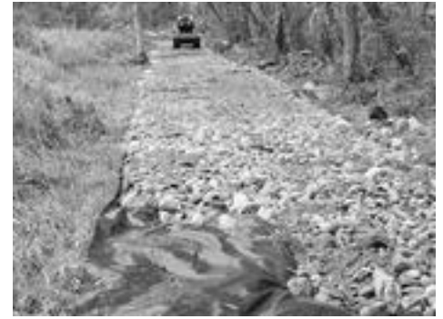
Improvements in progress along Springvale Farm Trail Photo: Jim Roux
