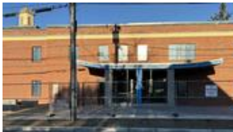
New Entrance to Goodall Library Photo: Lawrence Furbish
