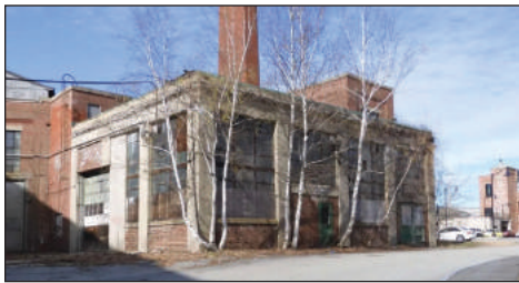
The boiler house of the International Woolen Company.
