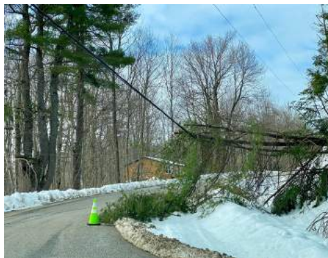
A limb is hung up on powerline three days after the storm. Photo: Tammy Wells
