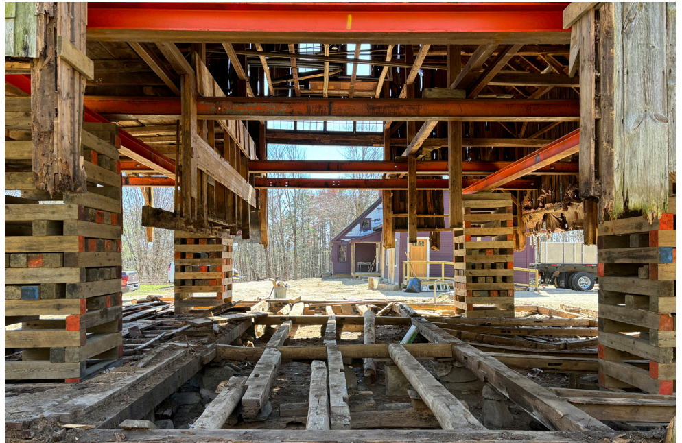
Ready for foundation work
